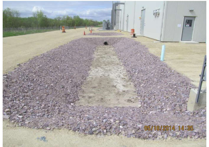
Installing site drainage west of electrical building
