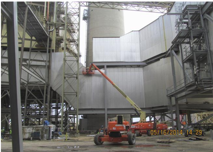
Ductwork tie-in on Unit 1 building
