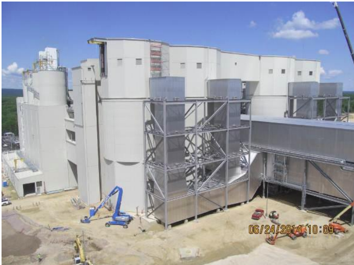
Overall construction looking northwest
