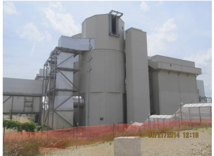
Overall construction looking southwest
