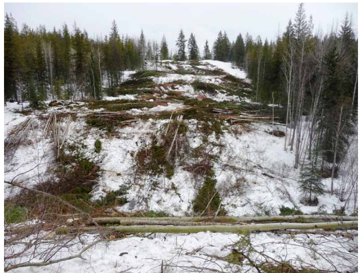
Right-of-way clearing for the new 69kV transmission line
