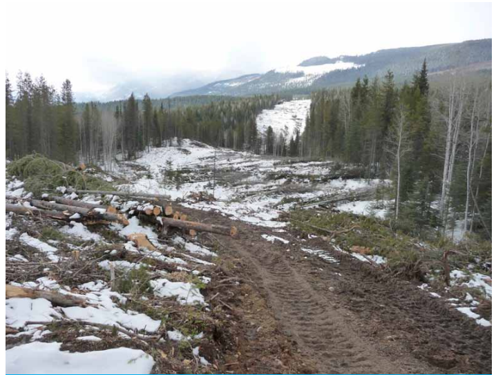
Right-of-way clearing for the new 230kV transmission line
