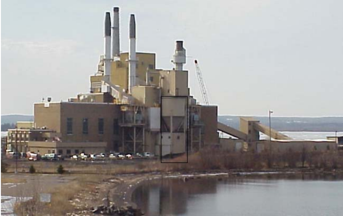
Figure 2. Eastern view of the Bay Front Power Plant in Ashland, WI. The baghouses and activated carbon injection systems will be located in the area of the existing ash storage hopper and enclosed ash unloading area (inside black rectangular box).
