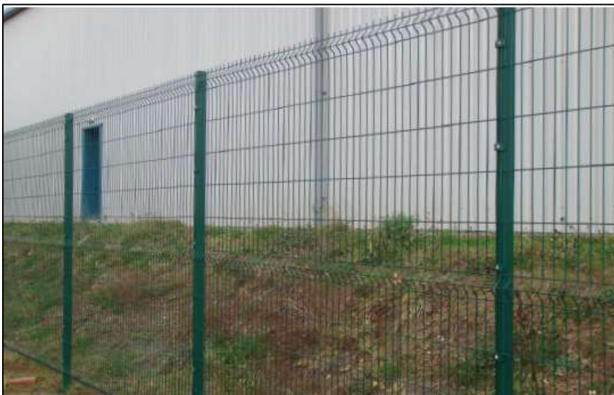
Picture: Typical fencing placed around the solar park
