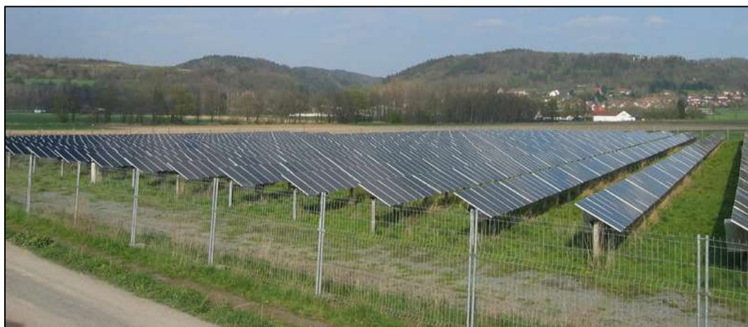
Picture: Module rows oriented towards South
