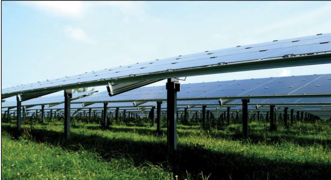
Picture: lower border of module table 80 cm above the ground
