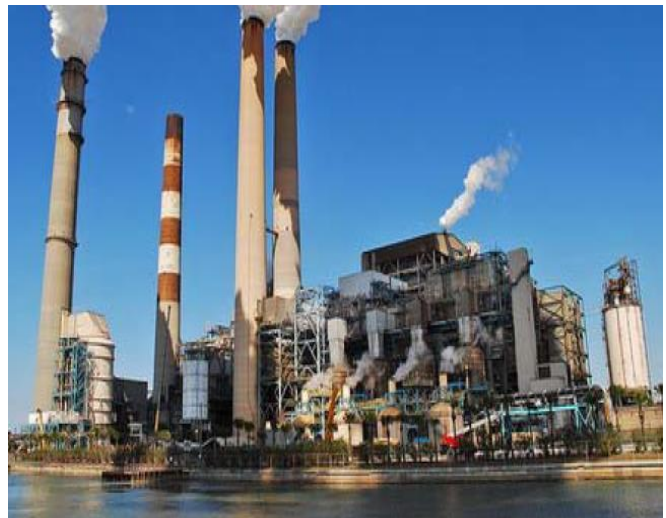
Figure 2. TEC Big Bend Station.
