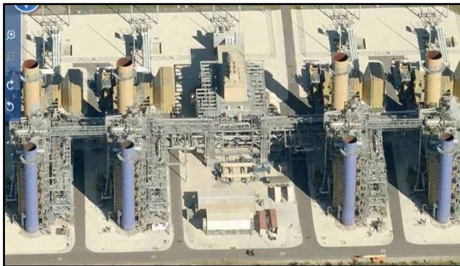
Figure 2. Duke P.L. Bartow Combined Cycle Unit 4 (~1,280 MW)
