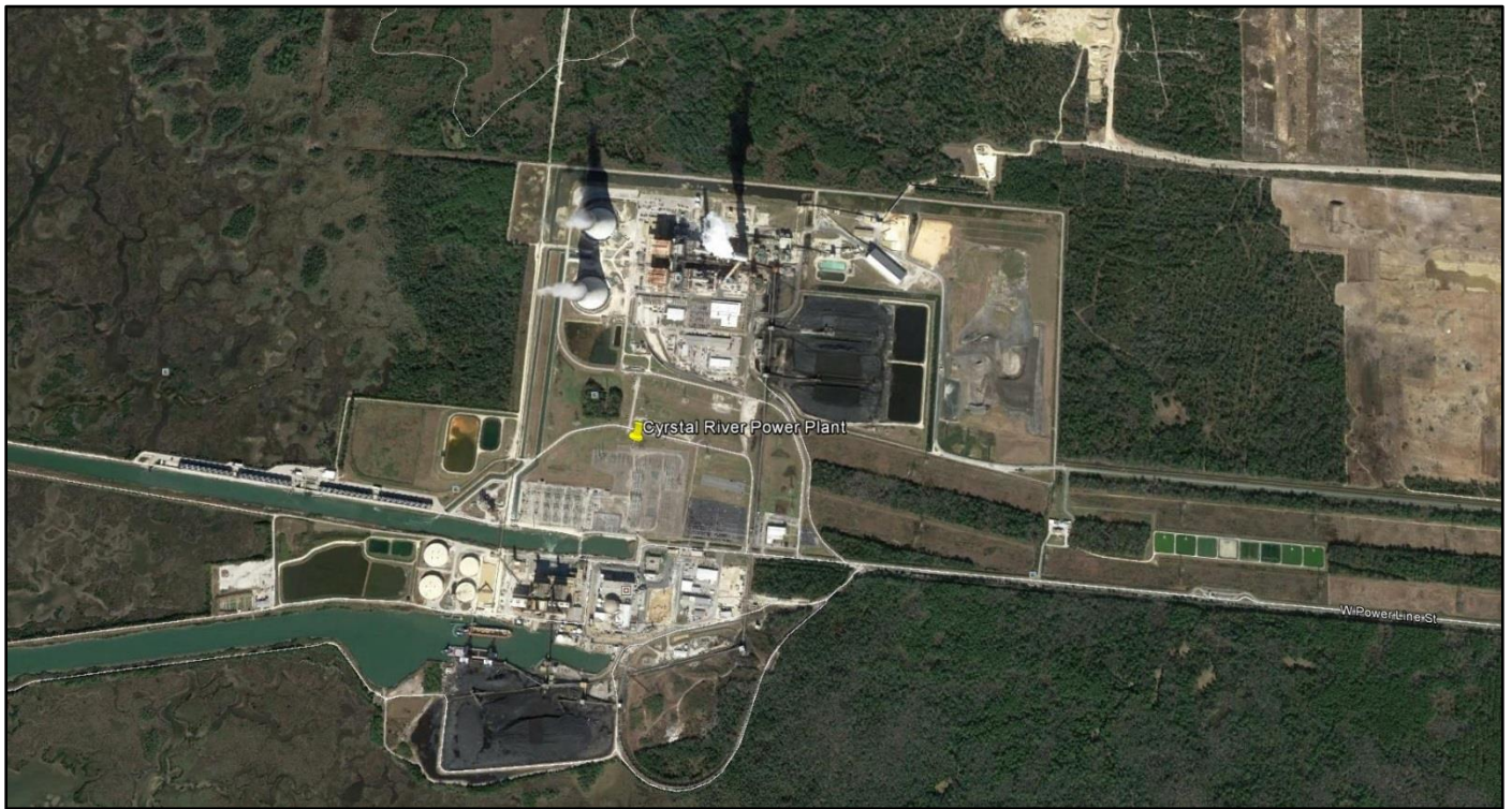
Figure 3. Satellite View of the Crystal River Power Plant.
