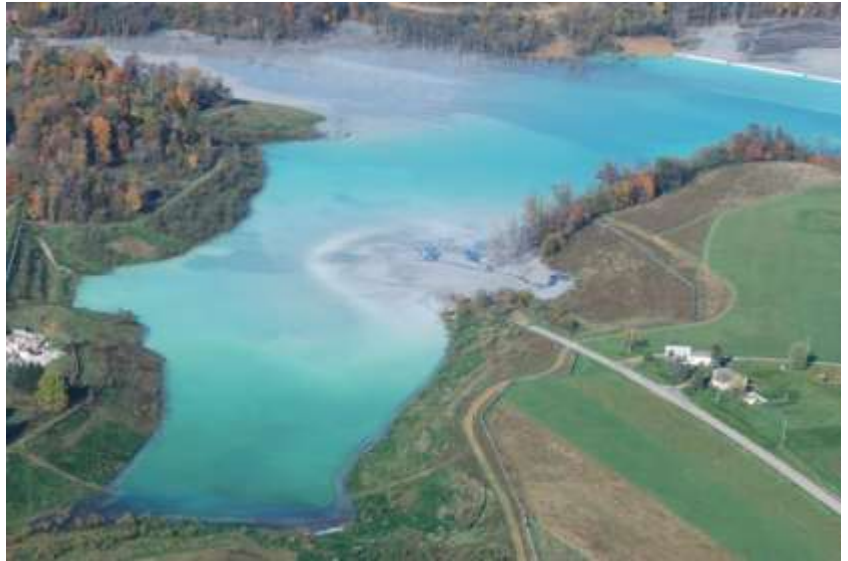
Nearly 1,700-Acre Little Blue Run Coal Ash Landfill in PA and WV (Oct. 23, 2011).
