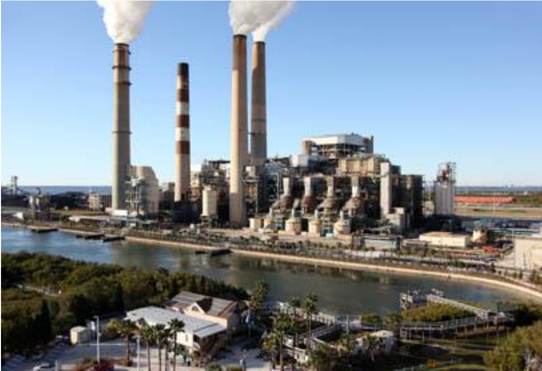
Figure 1. Big Bend Power Plant Showing the Unit 4 FGD for scrubbing Units 3 and 4 (bottom right, four scrubber modules seen to the right of all 4 stacks at ground level) and the new common FGD for scrubbing Units 1 & 2 (far left stack, FGD is connected at the base of the stack).
