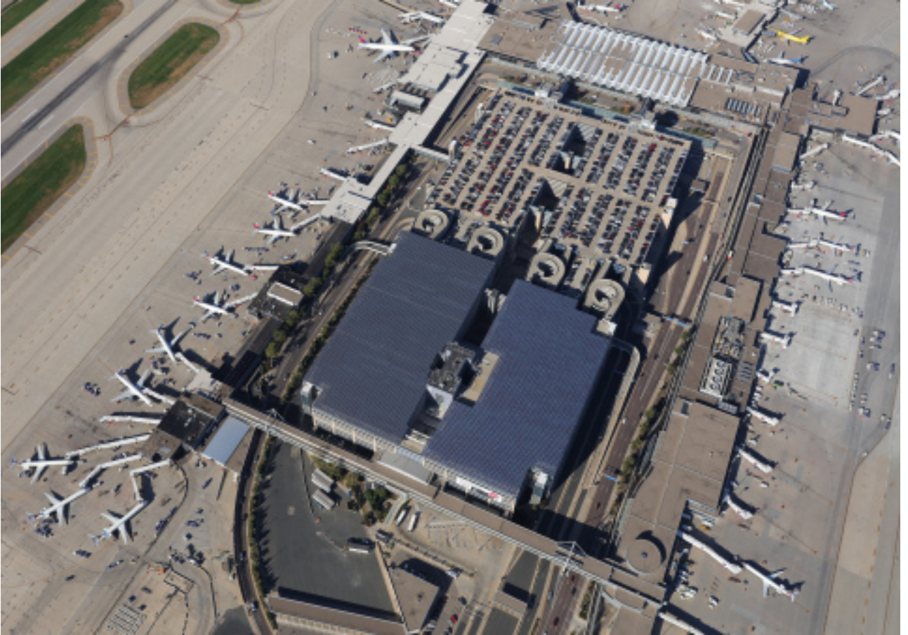
3MW solar installation on the top deck of two parking structures at Minneapolis-St. Paul International Airport.(Photo: Business Wire)
